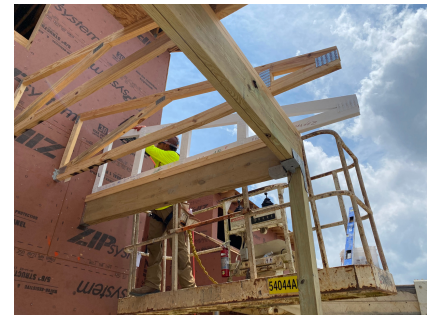
Dozoretz HHR Topping Off
